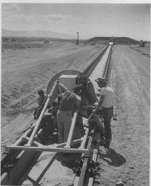
TEST TRACK shown here has rocket-propelled sled working in the picture are, L to R: Walter Drake,
